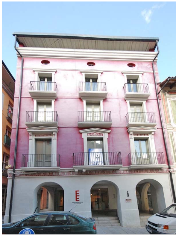
Façana Carrer Major (2015)
