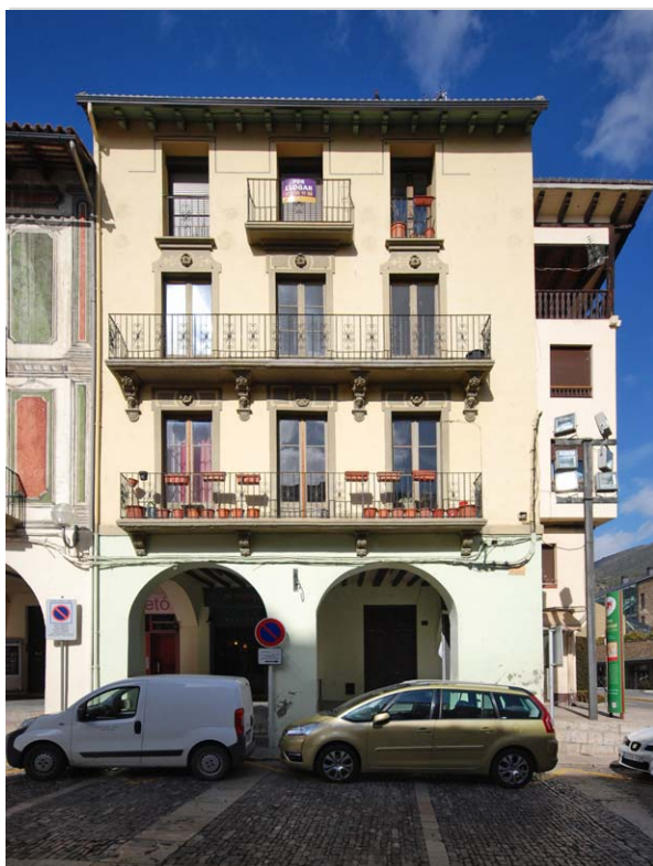
Façana Carrer Major (2015)
